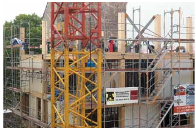
In future, timber-concrete hybrid constructions will become more popular
