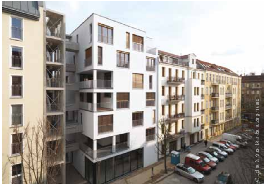
The fire engineering strategy for this residential timber building in Berlin was outlined
